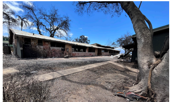
Wildfire damage to the original King Kamehameha III Elementary School campus.
