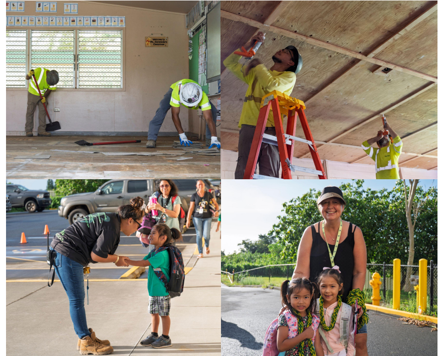
Top photos: Ongoing repairs at Nā'ālehu Elementary. Bottom photos: Welcoming Nā'ālehu Elementary students to the temporary learning site at Ka'ū District Gym.
